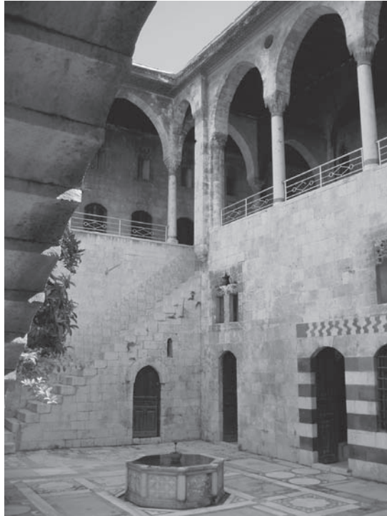
Figure 5.2 The house of Esad Pasha al-Azm in Hama, Syria ( c. 1740), showing both the Azm ‘trademark’ black-and-white striped masonry and the characteristic features of the courtyard house, discussed in Chapter 7.
